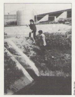
A pilot plant for treatment of night soil with anaerobic digestion, a biostabilization pond / fish pond.
