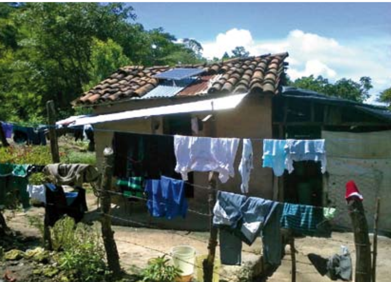
Female entrepreneurship benefits the whole family: from the daily chores to a rooftop solar system.
